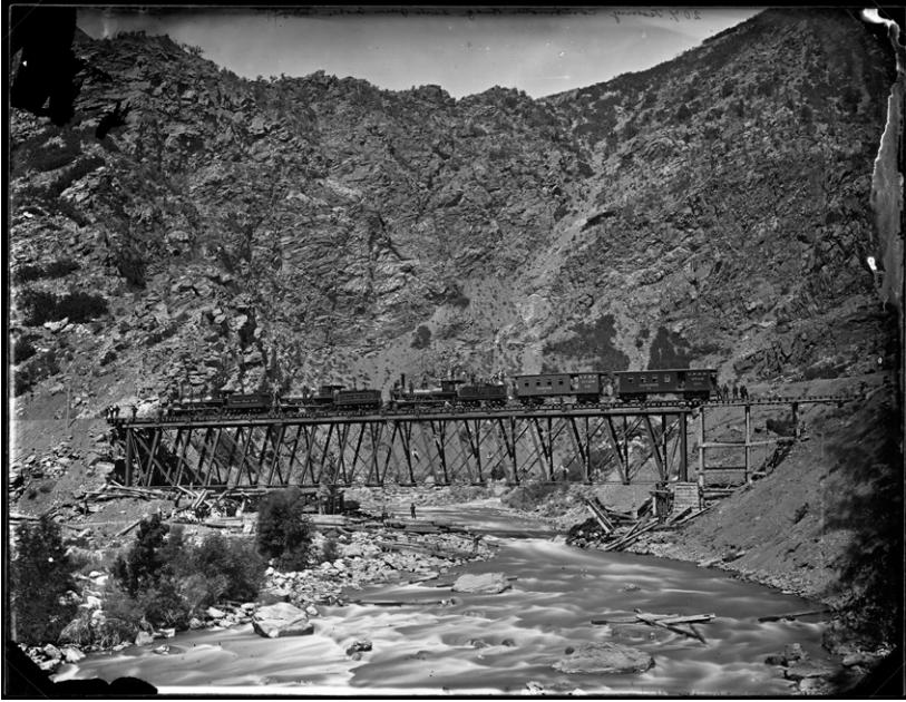
Russell, Andrew J. Testing Combination Bridge, Devil's Gate, Weber Canyon, Weber Canyon, UT. 1869. Imperial collodion glass plate negative. Collection of Oakland Museum of California.
