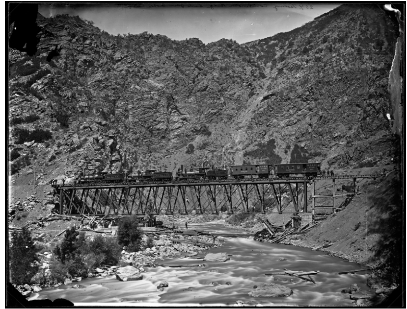
2. Testing Combination Bridge
