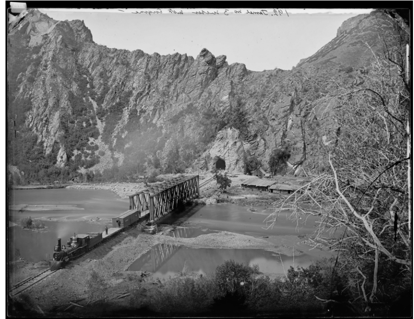
Russell, Andrew J. Tunnel No. 3, Weber with Engine . Weber Canyon, UT. 1869. Imperial collodion glass plate negative. Collection of Oakland Museum of California. http://picturethis.museumca.org/pictures/tunnel-no-3-weber-engine
